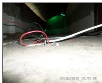
Photo of the inside of the main production hall NC B 11 6 4 Loose and joint wiring.JPG
